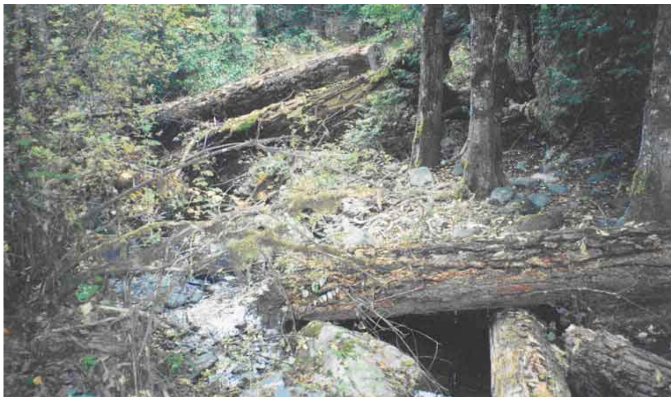
Catching Creek log structures
